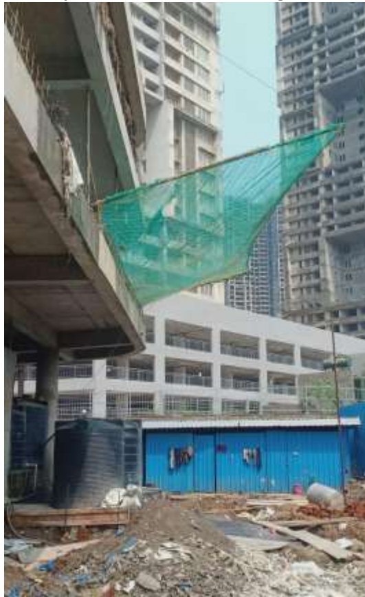
Safety Net installed
